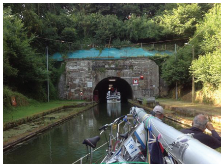
Tunnel S:t Quentin
